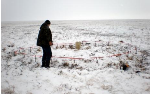
Preparation of CS grounding (grounded cable).
